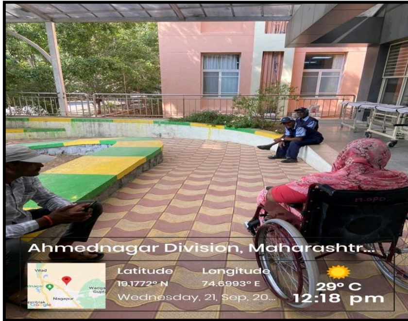
Ramp for Wheelchair and Stretcher
